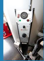
A pair of stand alone gas fired hot water storage units provide enough hot water for all the demands of the building. Water is stored at 65 Celcius to ensure any legionella bacteria are killed, the hot water is circulated throughout the building at 60 celcius preventing any bacteria surviving in the distribution pipework. Should one of these units fail, sufficient hot water is generated to meet the demand.
