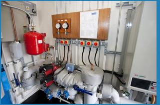
Three wall hung, fully condensing gas boilers are fitted. Controlled to operate on a cascade system maximising efficiency by supplying a "low loss header" pipework arrangement which only sends out the required volumes of water at optimum temperatures to satisfy the heating demands of the building. A boiler failure will not reduce the heating capacity ensuring continuity of service.
